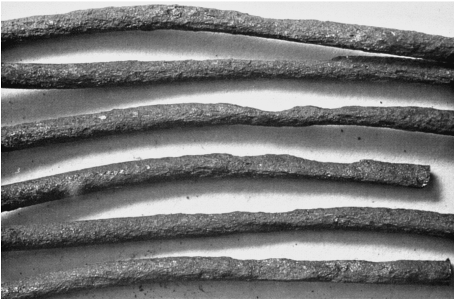
Figure A.7 — Corrosion excessive
