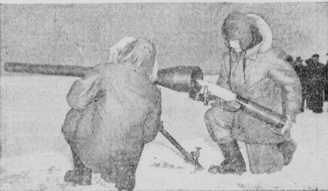
This unorthodox rifle developed by the United States Army weighs only 100 pounds but fires a shell capable of penetrating all but the most heavily-armored tanks. It is designed to give the infantry a readily portable gun capable of engaging and defeating armored vehicles. This Canadian Army photo shows Canadian soldiers testing the new weapon. (CP Photo)
