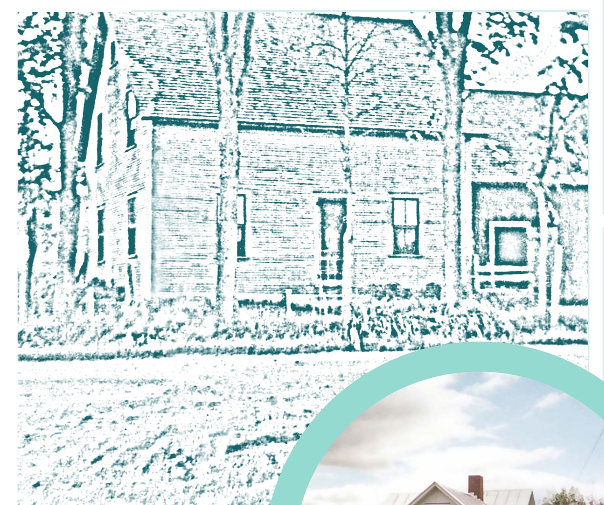
Mary Jane owned and occupied this house located at 1 Chemin Bice in Orford, from 1902 until 1919.
