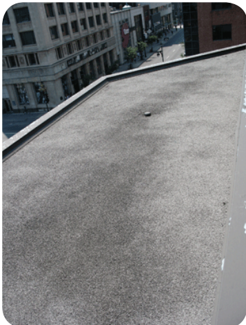
Image 17- Membrane multicouche, Pavillon Hubert-Aquin, UQAM
