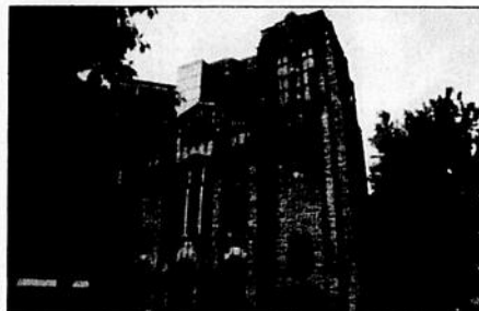
MONTREAL | PLATEAU $599,000 Unique and oversized residence within walking distance to everything! Former place of worship converted into luxury condos. 13 ft ceilings. Private terrace. A remarkable urban oasis. www.josephmontanaro.com
