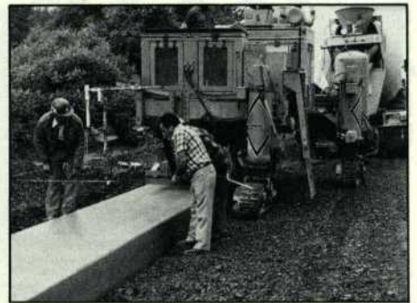
A Francon crew form a central mall with a Gomaco curb machine. Concrete is supplied by ready-mix units in the background.
