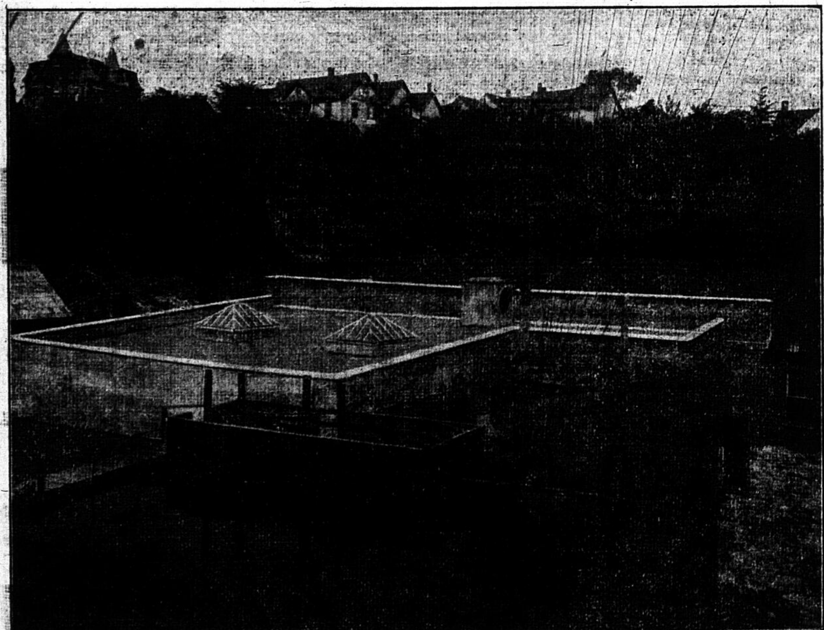
FIG. 2—VIEW OF NEW PLANT, SHOWING METHOD OF VENTILATION.
