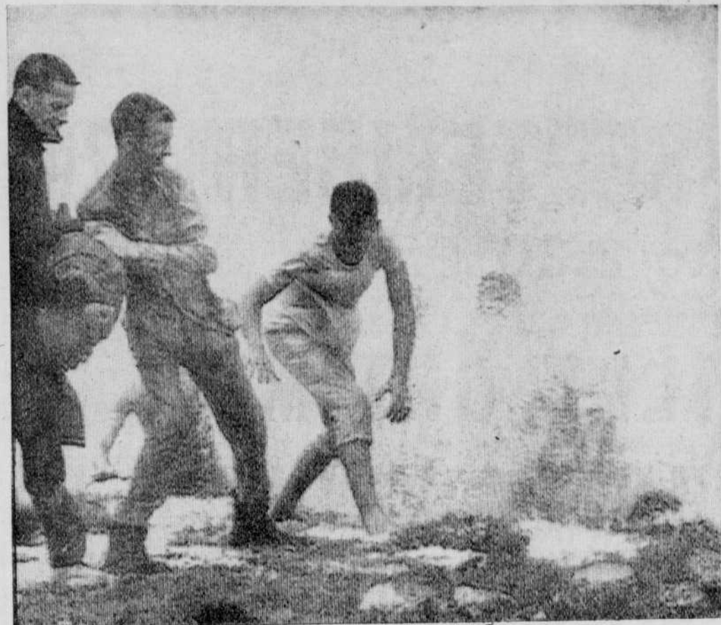
FIGHT DORA'S FURY — A group of volunteers pass sandbags and duck sea spray in an effort to save a seawall at Jacksonville Beach as the heavy seas and wind eat at the shore line. High seas have lashed the Florida coast and caused heavy damage to homes and power lines. (AP Wirephoto)
