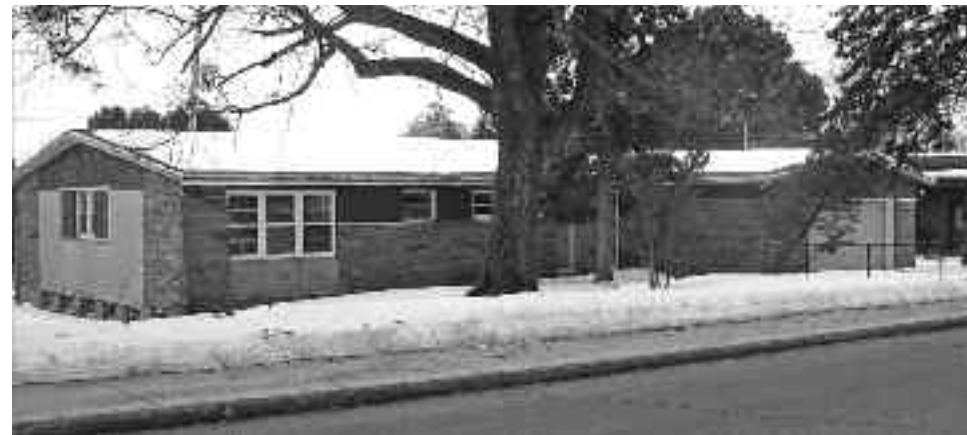
The existing bungalow at 4 Surrey Gardens.
