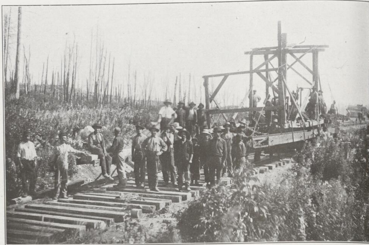
MONTREAL REACHES OUT INTO NORTHERN QUEBEC—Tie-laying at the rate of a mile a day on the Nominig-Rapide de L'Original branch of the C.P.R. (Photo by H. Richards.)
