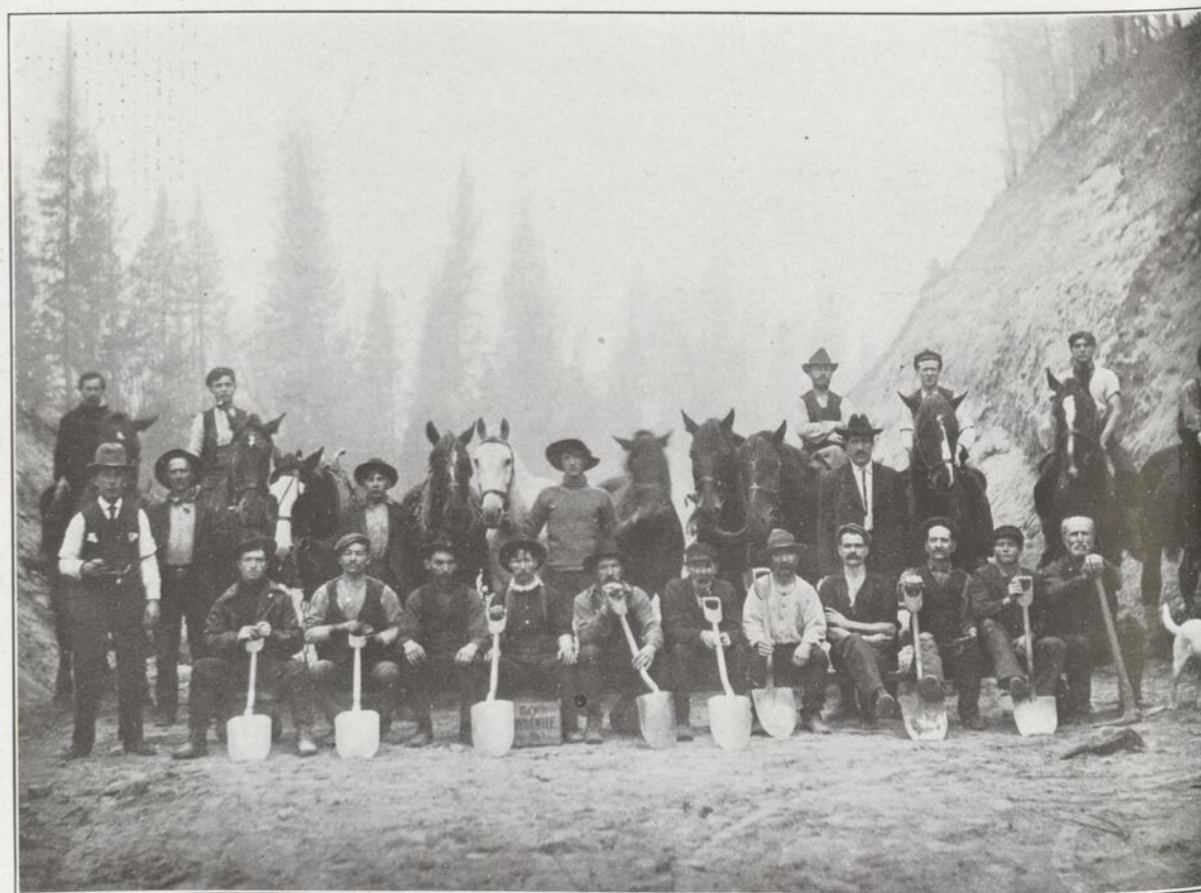
MONTREAL REACHES OUT INTO NORTHERN QUEBEC—One of the construction gangs on the Nominig-Rapide de L'Original branch of the C.P.R. (Photo by H. Richards.)
