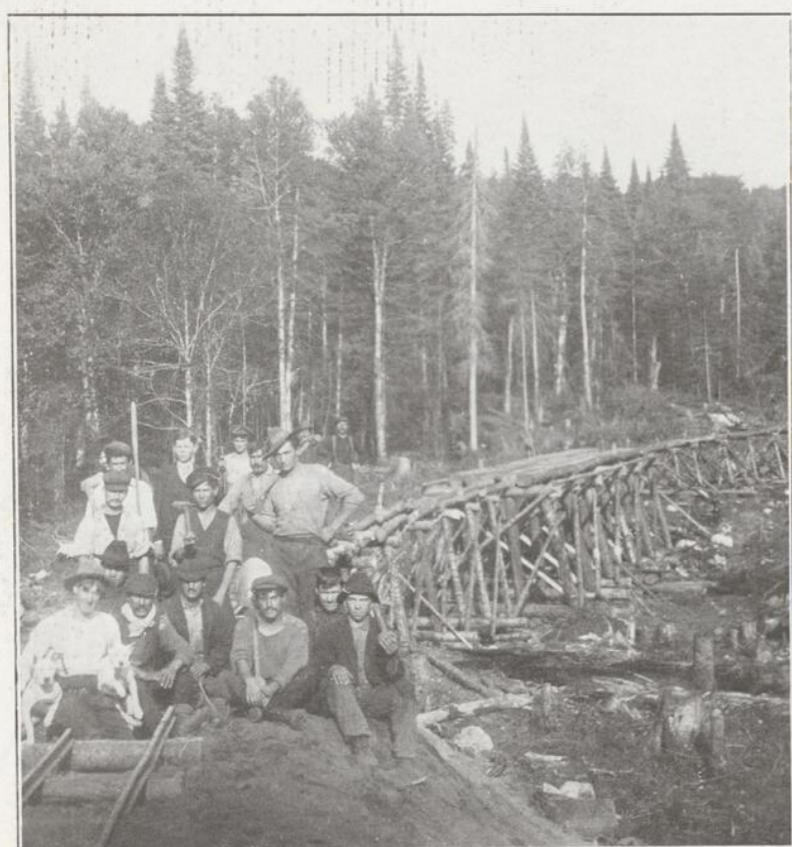
MONTREAL REACHES OUT INTO NORTHERN QUEBEC—Overcoming a swamp by trestle-work on the Nominig-Rapide de L'Original branch of the C.P.R. (Photo by H. Richards.)
