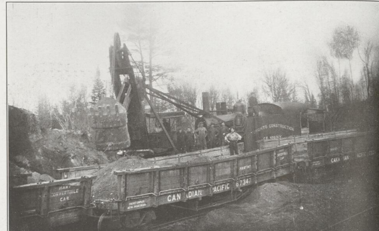
MONTREAL REACHES OUT INTO NORTHERN QUEBEC—A ballast train being loaded with gravel on the Nominig-Rapide de L'Original branch of the C.P.R. (Photo by H. Richards.)
