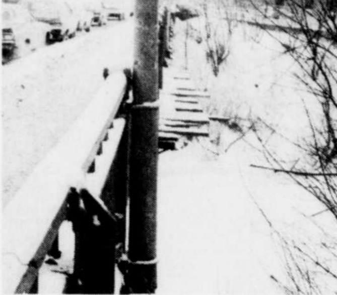
SUPPORT? — The rapid deterioration of the Wolfe Bridge is becoming increasingly more evident as winter continues to wage war on area roads and bridges. The stakes shown above are supporting the concrete sidewalk for a distance of 15 feet.
