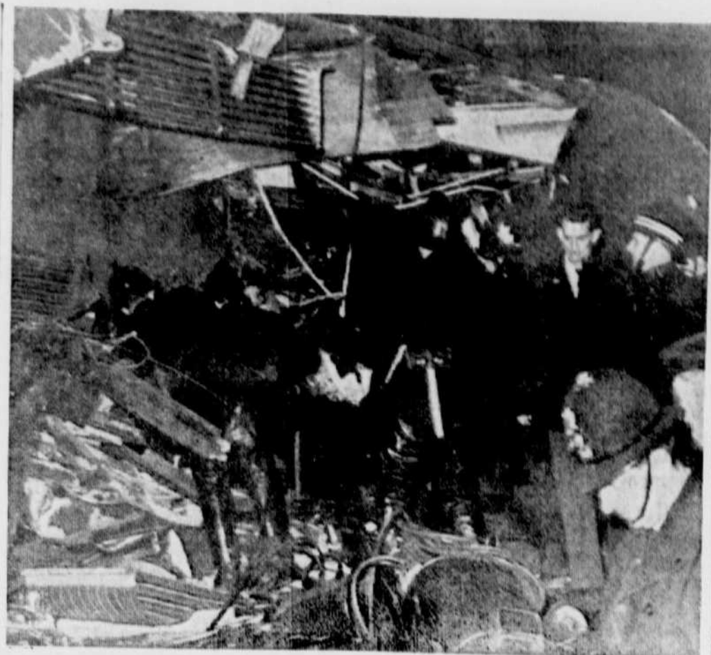
AFTERMATH ON WRECK — This was the scene Sunday night at Hither Green on the outskirts of London as police and rescue workers searched wreckage of crashed passenger train. The train jumped rails and overturned while en route from Hastings to London. Many casualties were reported. (AP Wirephoto via cable from London)
