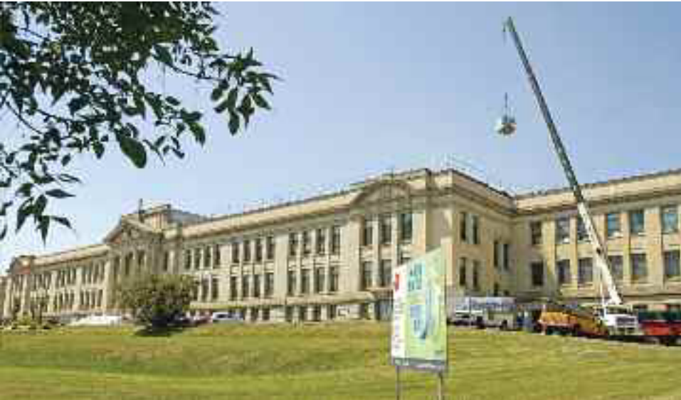
Crane at work at Marianopolis on August 8.
