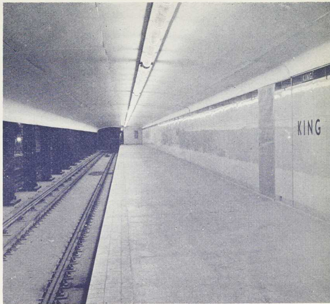
Partly Installed Station Finish — Toronto Subway
