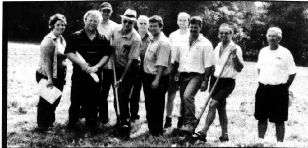
Hinchinbrooke Mayor Normand Crête recently turned the first sod for the new municipal fire hall in Athelstan. The new station will include a three-bay garage as well as a fireman's meeting room and a chief's office. The new station will replace the old station across the street in the town of Athelstan, which is no longer adequate. At the same time, the architect, engineer, contractor, municipal employees and some councilors and firemen were on hand (above) to decide the location of the new building. (Source: Carolyn Cameron)
