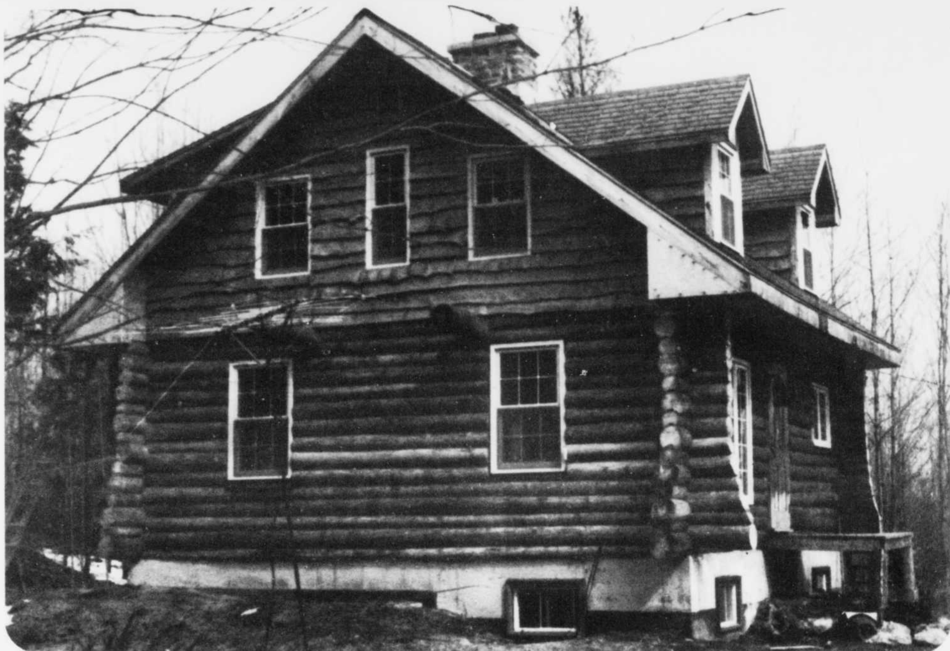
John Mines' log house in Abercorn is an example of the pioneer type buildings that are popular in Canada today.
