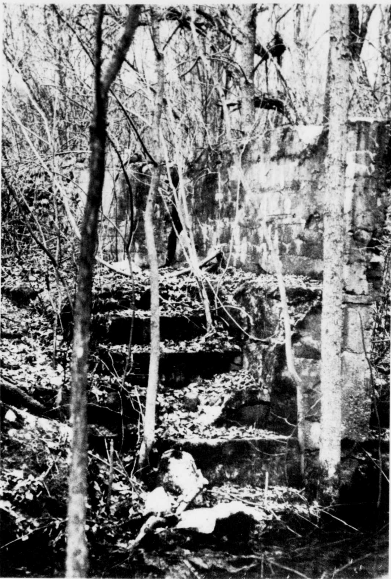
Falling walls and moss-covered rocks are all that remains of North Hatley's dam on the Massawippi River. Built in 1898, it produced electricity for North Hatley, Waterville, Compton, Eustis and Capleton. But, in those days, electricity only meant lighting.
