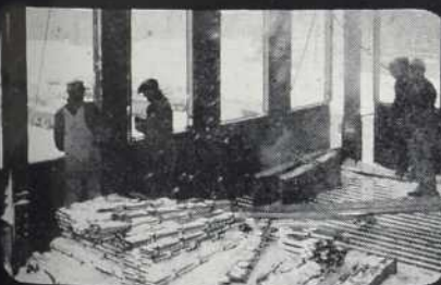
All weather construction
