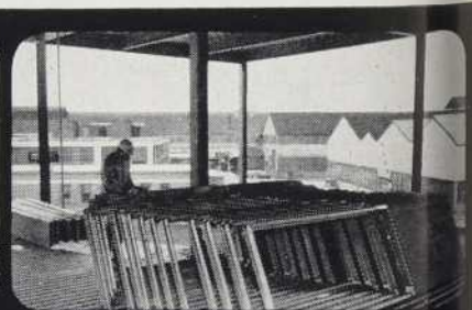
Panels stored within structure
