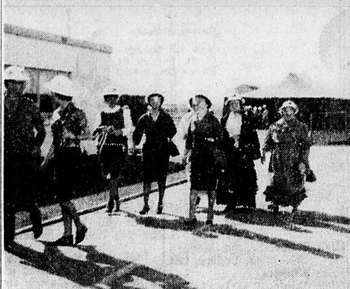
On the occasion of Beauharnois Centenary Celebrations, Standard Chemicals Ltd., invited the public to visit their plant on Sept. 25. All visitors received safety helmets. Above we see some of the main phases of the work done at Standard Chemical Ltd. Guides were furnished for the more than 500 persons who visited the firm. Mr. A. H. G. Sturton, manager of the plant, welcomed the visitors. Right, a guide explains the various phases of the work done at Standard Chemical Ltd. Lower left: Group of eight persons at a time visit the plant, you will note some of the people wearing 1863 costumes. Lower right: we see some of the guests eating the tasty refreshments provided for them on the course of the afternoon.
