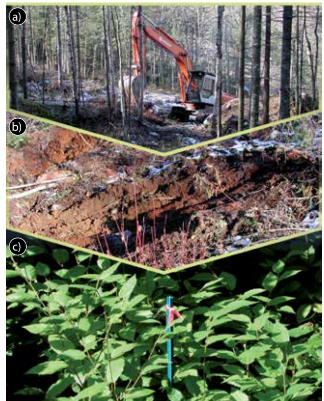
Figure 23. Spot scarification was performed by an excavator (a) to produce 1 m x 2 m spots (b) with the goal to establish yellow birch regeneration (c). Photos: Daniel Kneeshaw (a, b) and Patricia Raymond (c).
