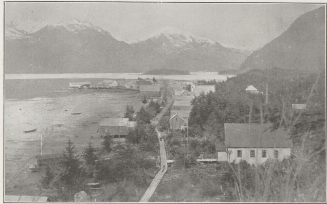
A PACIFIC CITY BUILT ON STILTS —View of the approach to Essington, British Columbia, a city that enjoys the distinction of being built in a manner quite different from other Canadian cities.
