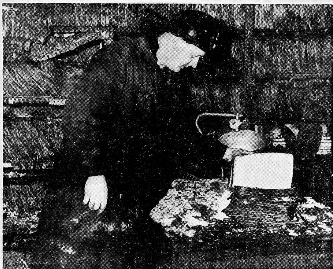
A Westmount fireman inspects the records room of the Reddy Memorial Hospital following the blaze which started in the hospital Sunday. The origin of the blaze is still unknown, Chief
