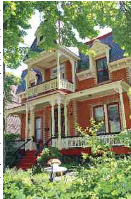
Two mature maple trees stand in front of this 1894 turreted home in Westmount's southwest.
