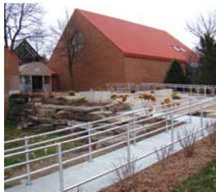
Borough Hall's West entrance is now accessible for persons with reduced mobility.
