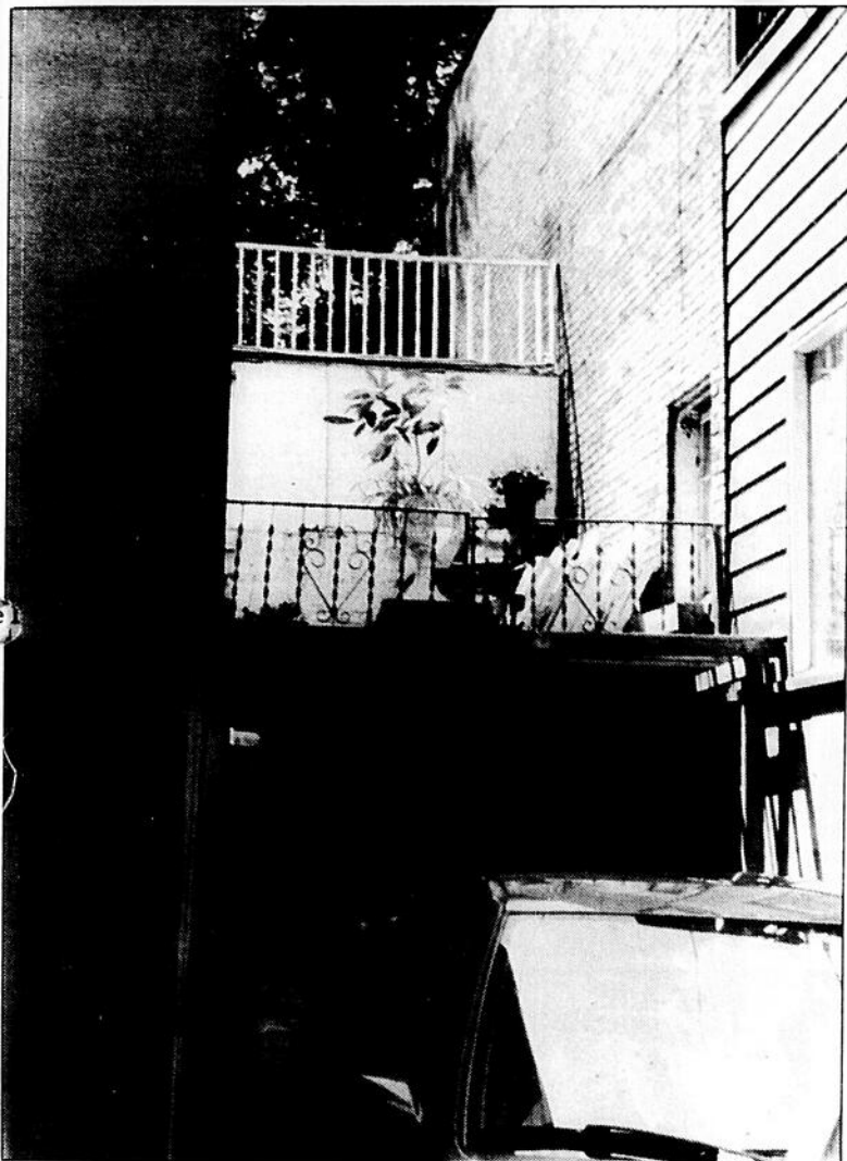
A controversial carport and sun deck behind 3 Prospect St. are the crux of a neighbours' dispute that first hit the courts in 1989.
