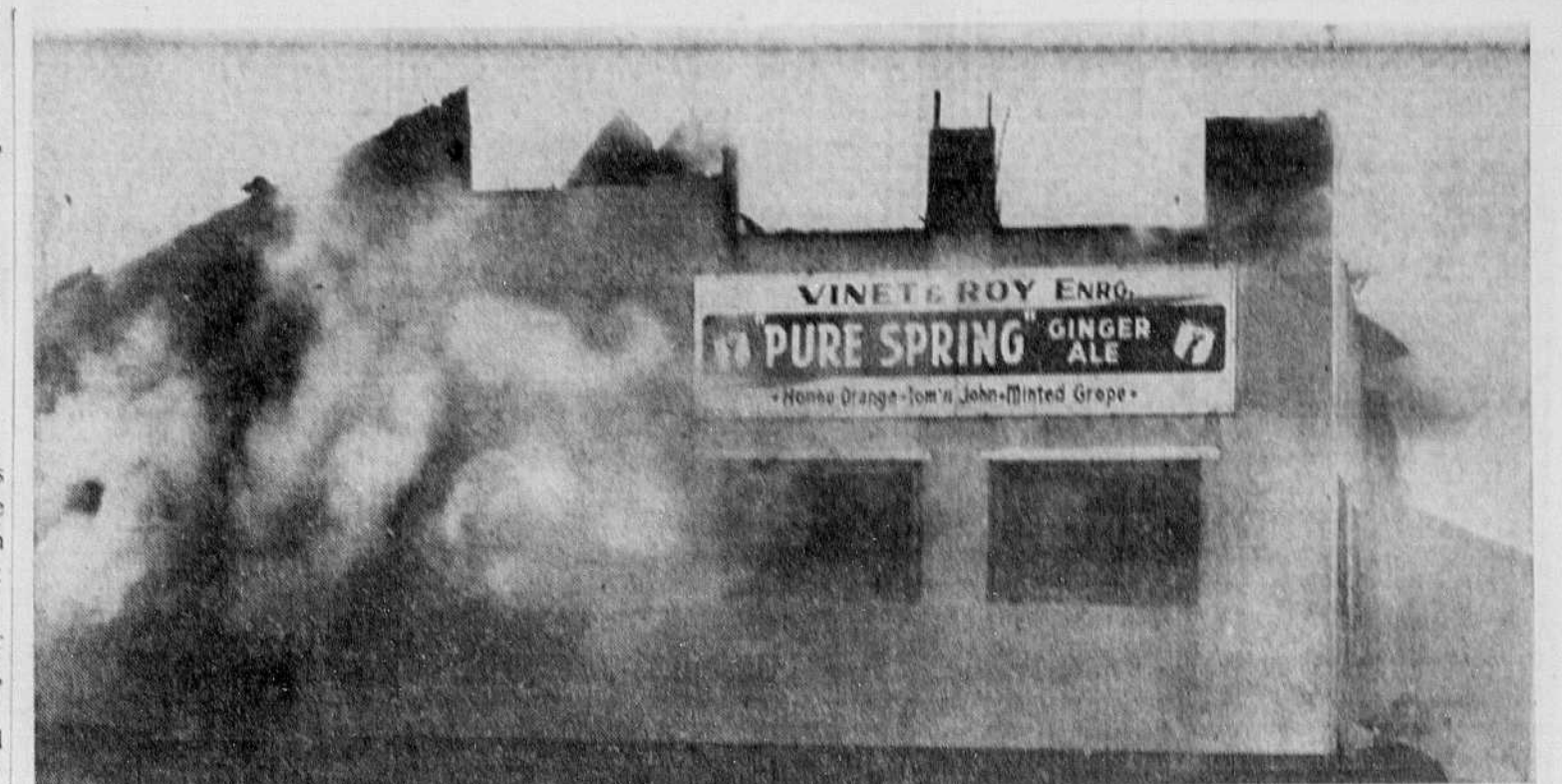
BOTTLING PLANT BURNS — Flames, fanned by a brisk wind, tore through Pure Spring soft drink bottling works on Galt St. West this morning and at press time firemen were pouring gallons of water on the ruins.
