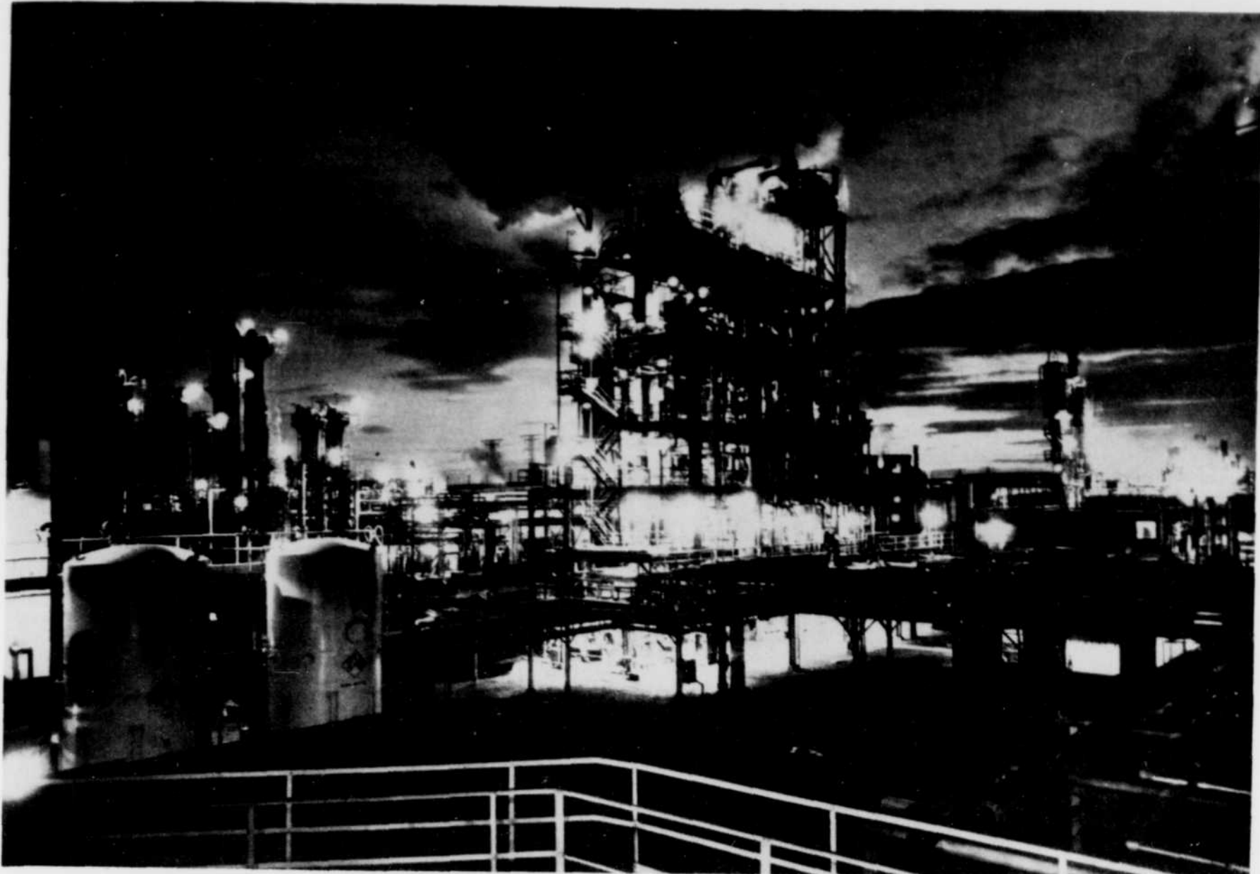
PLASTIC WORLD — Union Carbide Canada Ltd. has completed a $5.5 million expansion at its Montreal East petrochemicals complex. The project includes new facilities for the refining of propylene at rates in excess of 100 million pounds a year and permits an expansion of the plant's existing polyethylene capacity by 50 million pounds to 200 million pounds annually. Propylene is
