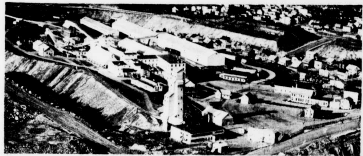
Above, a birds-eye view of the imposing Bell Asbestos Ltd. in Thetford Mines. In the background a partial view of the City of Thetford Mines.
