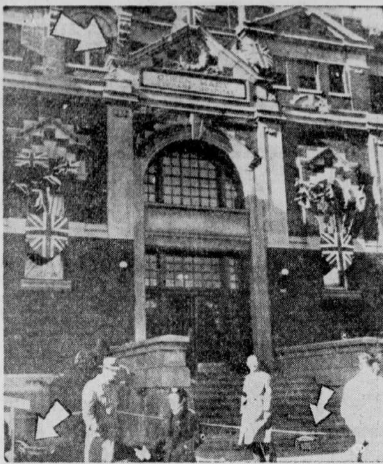
NEAR TRAGEDY —An accident came close to marring the last of the functions arranged for the tour of Montreal by Princess Elizabeth when a chunk of concrete crashed to the veranda of Queen Mary's Veterans' Hospital close to where the Princess had been standing. Arrows point to the cornice from which the piece of masonry fell and (bottom) the chunk of concrete and the flag in the ground at the front of the hospital. The Princess had moved from the spot about a minute before the masonry fell. (CP Photo)
