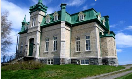
Old Law Court building in Kamouraska
