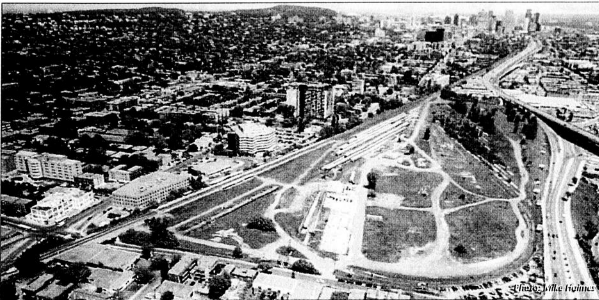
Aerial view of the Glen Yards, site of the proposed MUHC superhospital.
