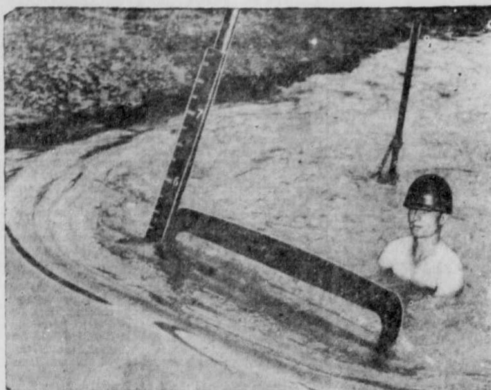
DEEP-SEA DRIVER — Pvt. Malcolm D. Zahary, Houka, Miss., proves that it's no trick to drive a Jeep through five feet of water. The demonstration is part of an Army course in readying vehicles for fording rivers. Zahary is an instructor at the Automotive Maintenance School, Fort Chaffee, Ark.
