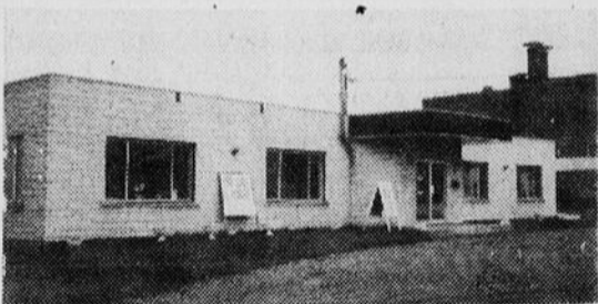
1) BEAUHARNOIS: Excl. Commercial building, ideal health center, 7 to 11 convenient store, medical center, lakefront, electric heating, available at once, will consider any offer. Marcelle Beaulieu 691-7030 or 691-2768
