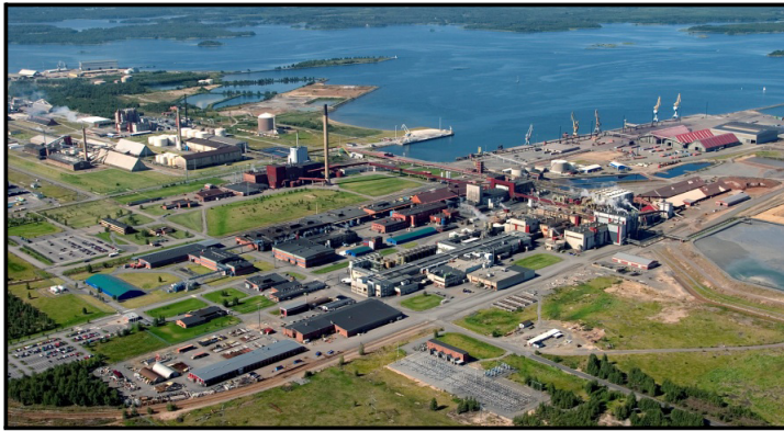
Figure 5.21: Kokkola Zinc Works.
