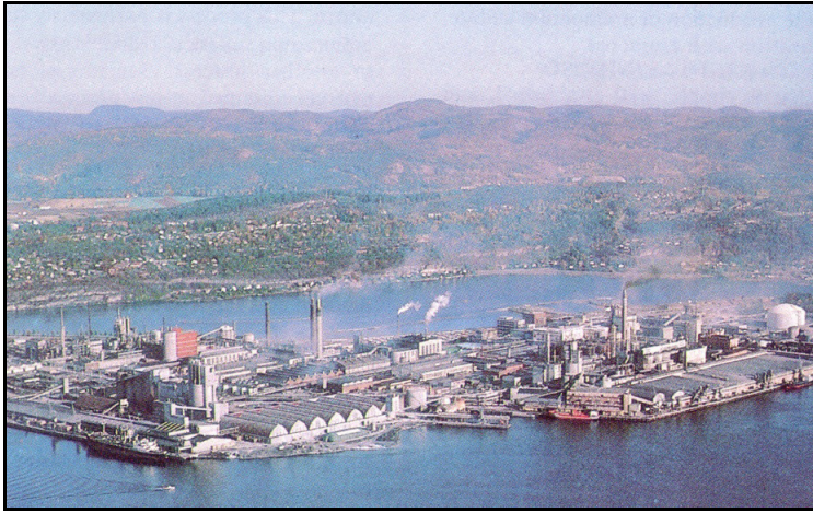
Figure 3.30: View of Porsgrunn Norsk Hydro plant.
