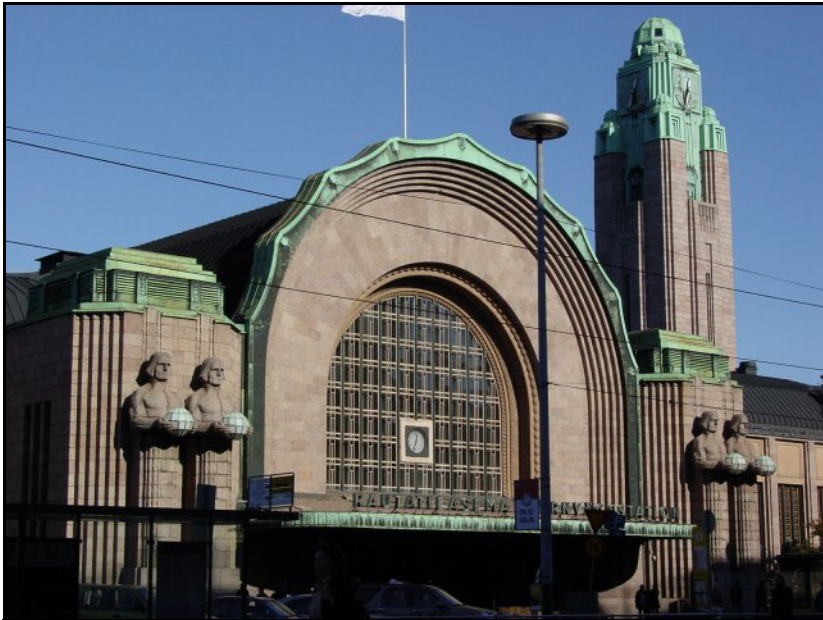
Figure 5.6: Helsinki Railway Station.
