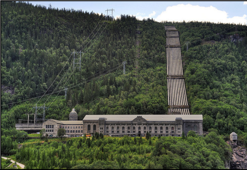
Figure 3.28: Ammonia synthesis plant showing the pipes carrying the pressurized solution to the top of the mountain then descending to drive the Pelton wheel to recover the energy.
