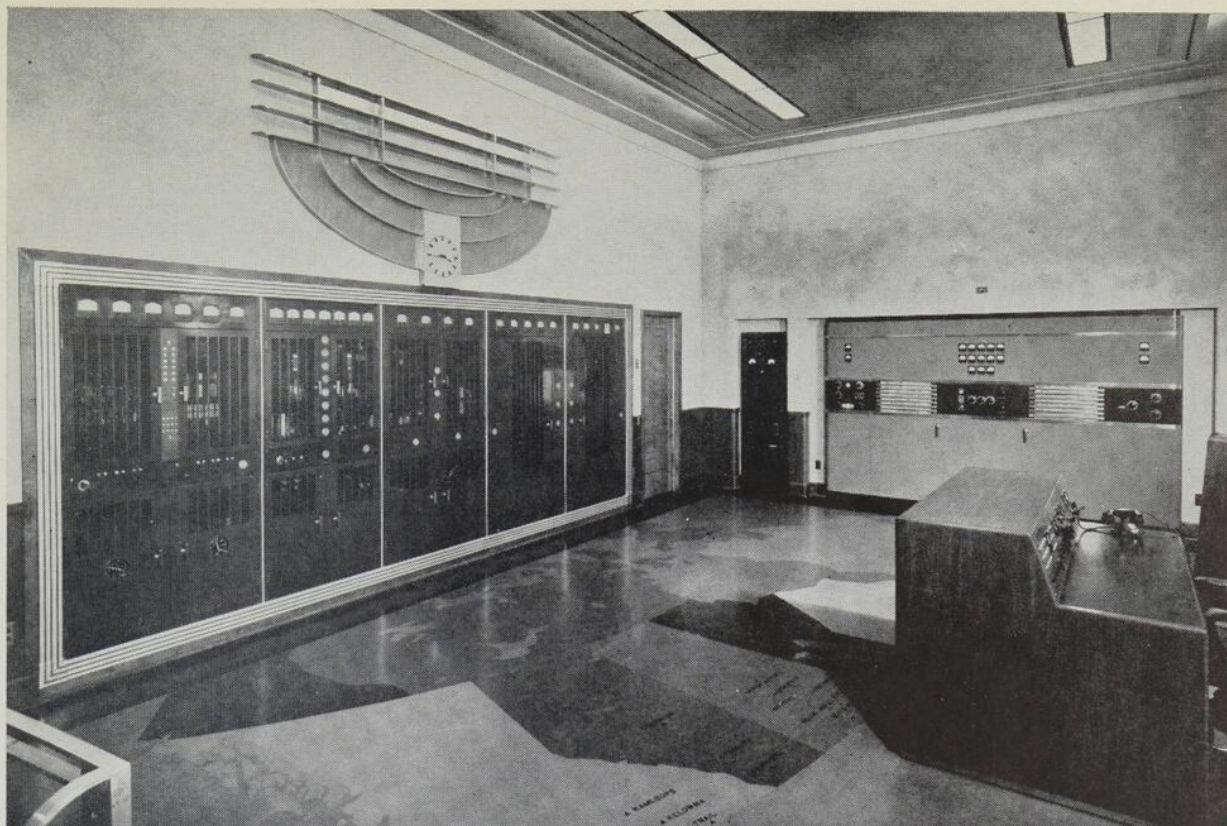
Interior view of transmitting station CBF, CBFY, CBFW of the Canadian Broadcasting Corporation.
