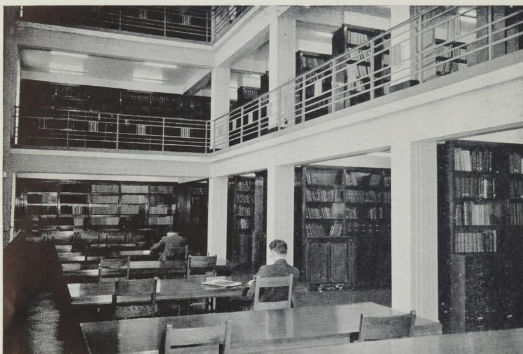
The Library of École Polytechnique — Main lecture room.
