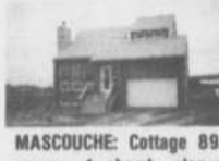
MASCOUCHE: Cottage 89, garage, 4 chamb. plaque chauff. Four encastré, foyer terr. 9,051 p.c.
