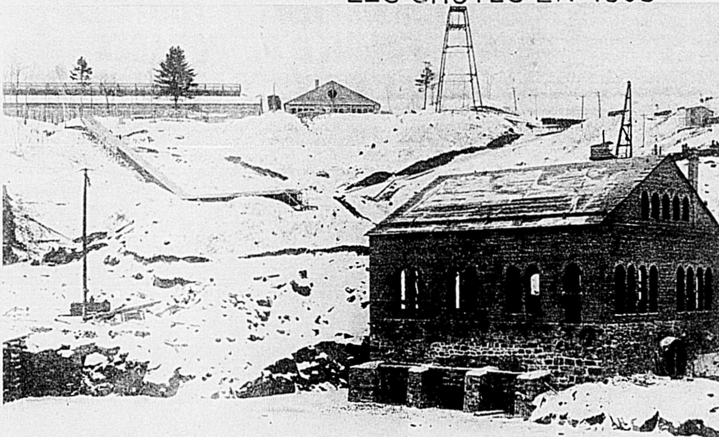
LA CENTRALE DE LA PITTSBURGH REDUCTION 1900
