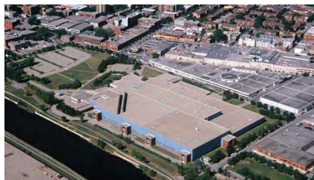
Former Canada Post mail sorting facility on the north bank of the Lachine Canal
