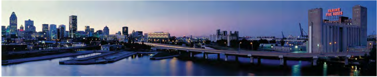
Night view of Peel Basin and Bonaventure Expressway seen from the Cereal Foods Canada silo
