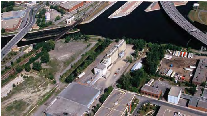
The filled-in site of the former Tate and Wellington basins
