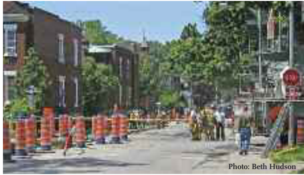
Looking north on Prince Albert at Somerville, July 3.
