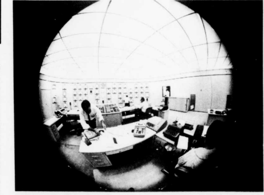
The output of a number of electric power generating stations is controlled from a central room by this small group of operators.
