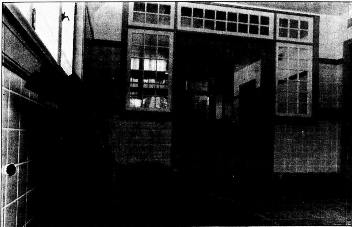
The newly renovated comfort station in Westmount Park opened last week to the tune of $118,000 worth of new features, including a new heating system and handicapped access. Benches are on the women's and men's sides, with a common area and large windows between.
