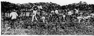
Digging asphalt from Trinidad Lake for Genasco
