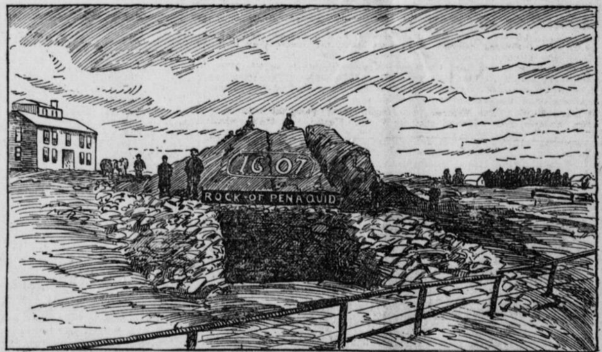
WHEN THE EXCAVATIONS WERE BEGUN.
