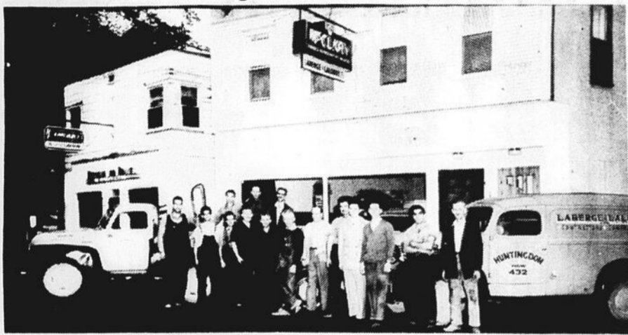
This is the Loberge and Lalonde Plumbing and heating contractors in the early 1950's where Mon Boucher is located today. Next door was the S.J. Currie Electrical Shop. Pictured are from left: Ronnie Lalonde, George Lazure, René Legault, Harold "Jake" Higgins, Euclid Loberge, his brother Alec, Gerry Lalonde, Irvin Loberge, Roch Dumouchel, H. Faubert, Paul Forget, Johnnie Hurteau, (rear): Paul Lazure, Tommy Finigan, and Charlie Lazure.
