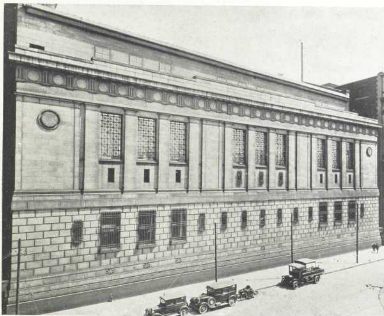
Bank of Montreal, Craig St. Elevation (1903) McKim, Mead & White, Architects
