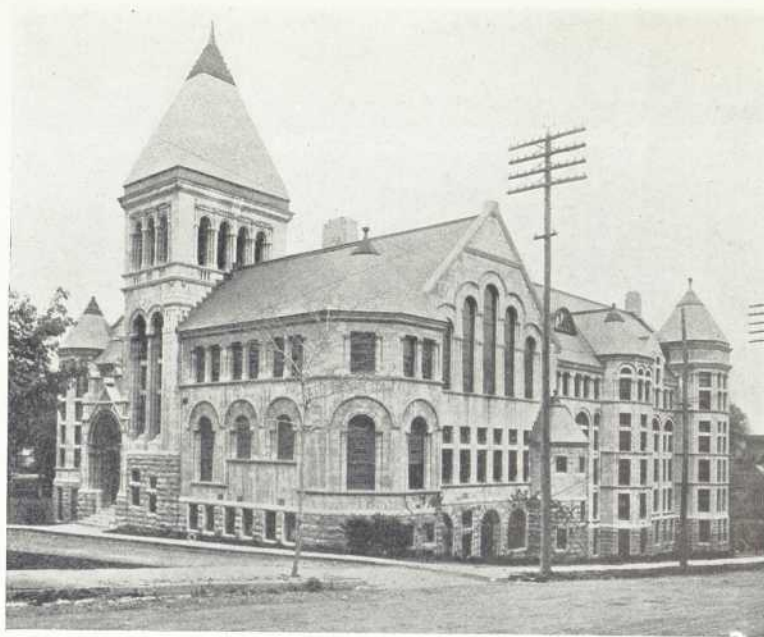
The Library, McGill University (1891) Taylor & Gordon, Architects
