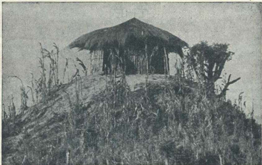
Hut constructed over an anthill.
