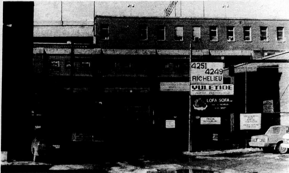
Viewed from Richelieu street in St Henri, this warehouse is recessed behind others and located over the border in Westmount.
