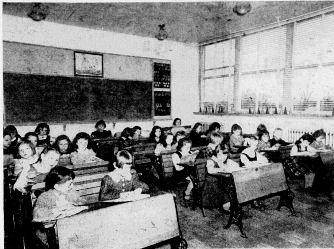
Above is a typical classroom in the new Notre Dame School, Huntingdon, showing the tiled floor, large amount of window space, the vestibule blinds and the "musite" blackboard which is made of glass and is green in colour. A somewhat different style of desk is used in this room to most of the classrooms in the school.
