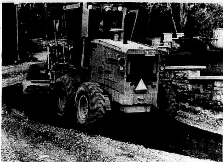
Construction crew smooths gravel along Belvedere Rd.
