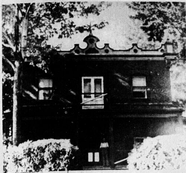
APPOINTMENT OF Jules Léger as Canada's new governor-general has aroused interest in two old buildings in St. Anicet where the Léger family resided. One is the old Léger homestead (left) and
