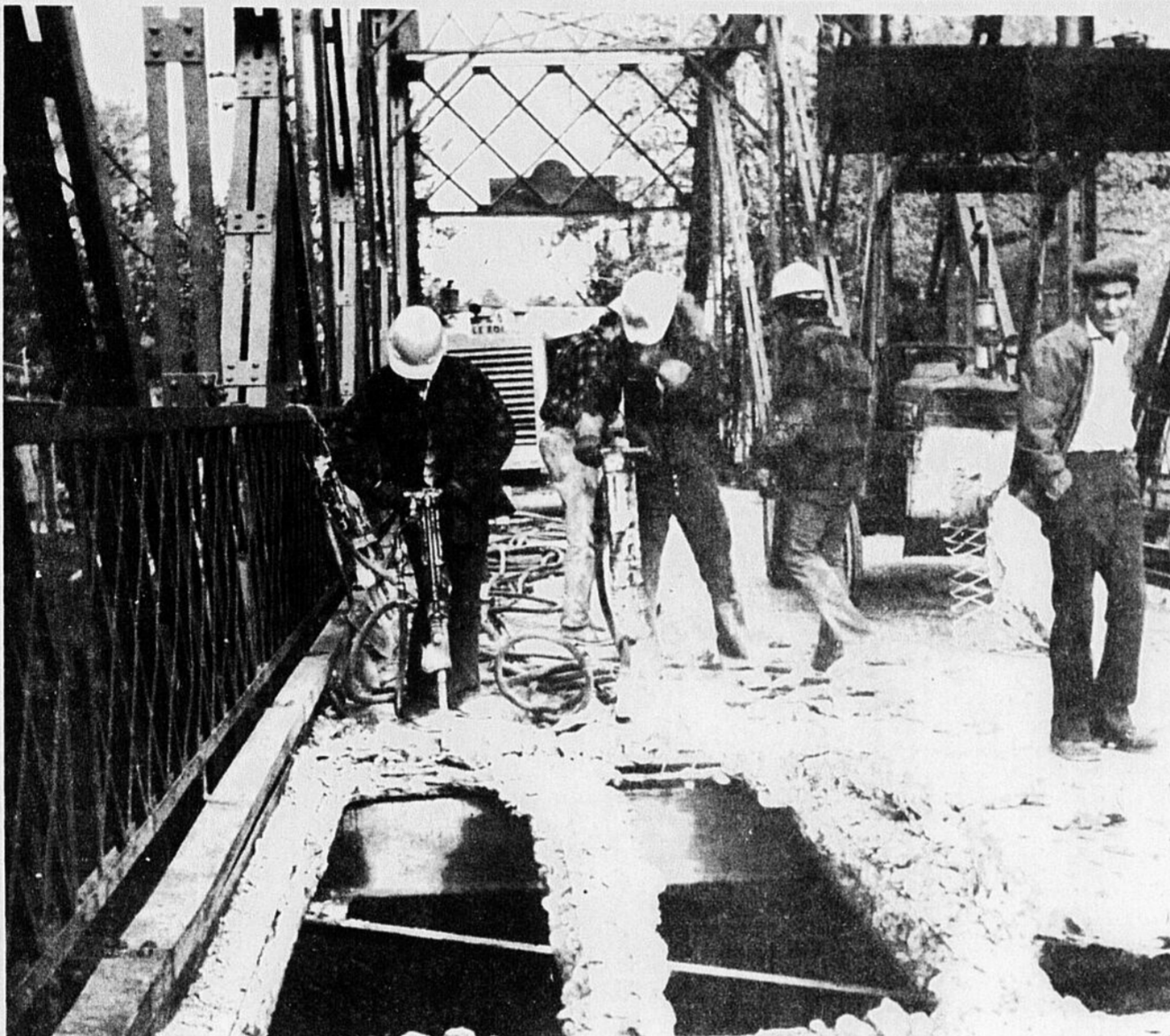
THE ROADWAY AND SIDEWALK of Walker Bridge in Huntingdon are finally being replaced. Citizens had long protested against the holes through which could be seen the rushing waters of
