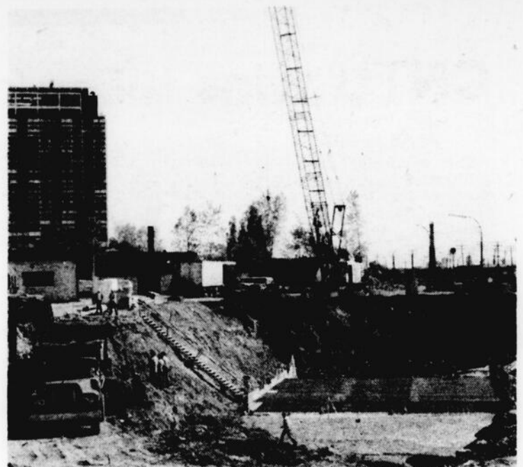
CONSTRUCTION STARTED: Construction of the Vendôme Métro station, just past Westmount's western border, now is well under way and should be completed within two years. The station will serve Westmount's CPR station, the Queen Elizabeth Hospital and nearby commercial and residential establishments, including the offices and apartments of Château Maisonneuve, at upper left of photo.
